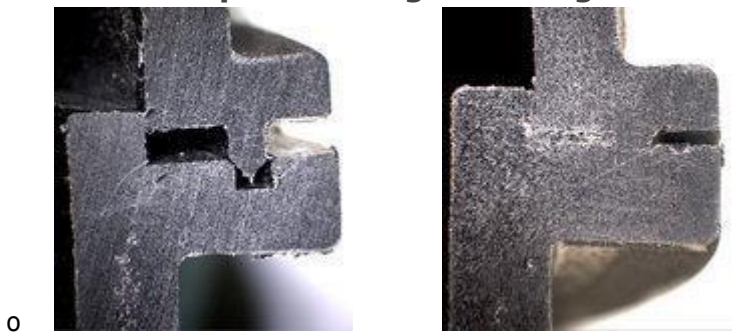
o Unwelded condition Welded condition
